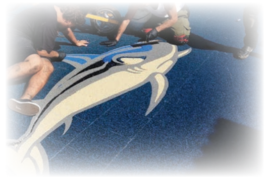
Wear Course (1/2" EPDM Top) Cushion Course (Varying Depths depending on your fall height requirement) Sub-Base
