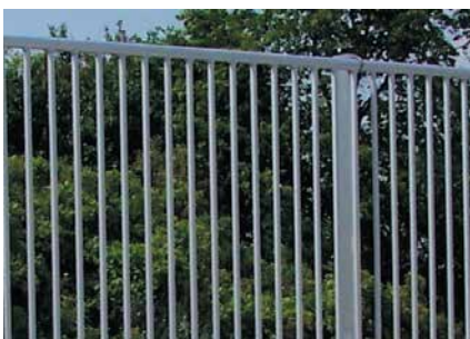
VERTICAL PICKET GUARDRAIL SYSTEM
