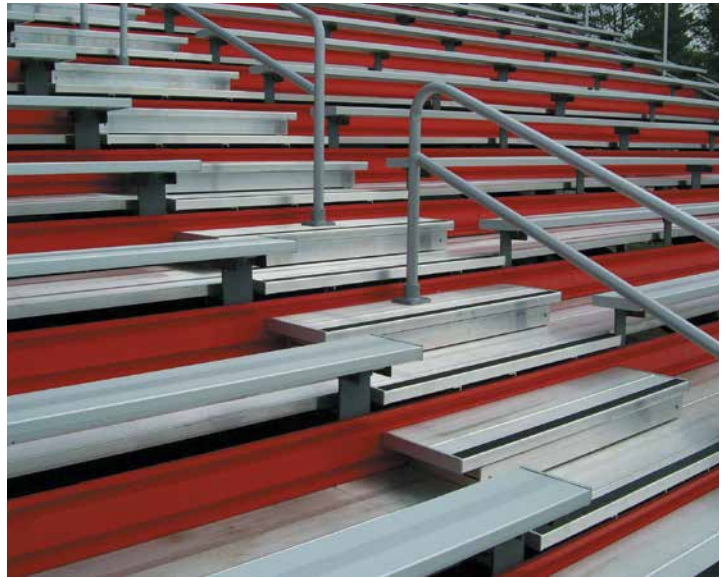
ALL OPENINGS CLOSED TO LESS THAN 4" FOR COMPLIANCE
