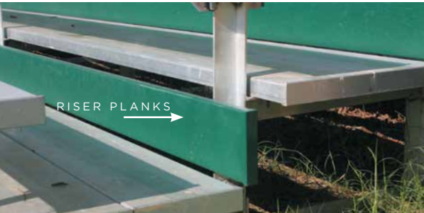
RISER PLANKS ON ALL ROWS
