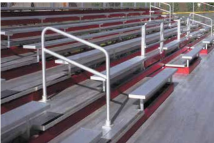
AISLE WITH HANDRAIL
